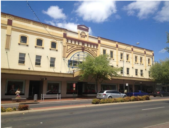
PICTURE 1 – LATE 19 TH CENTURY FAÇADE ON SUMMER STREET.
